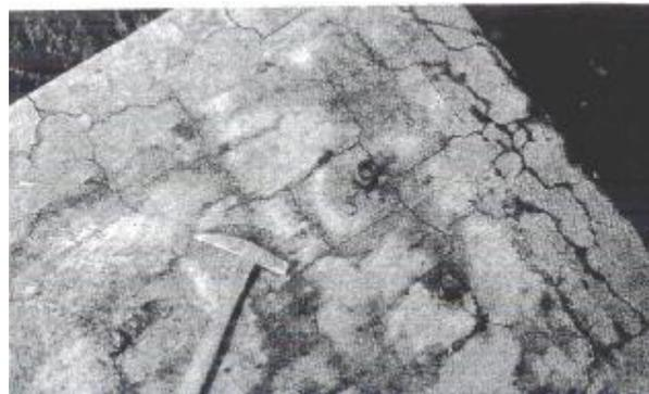
Fig. 4.1, Deterioration From Alkali-Silica Reaction
